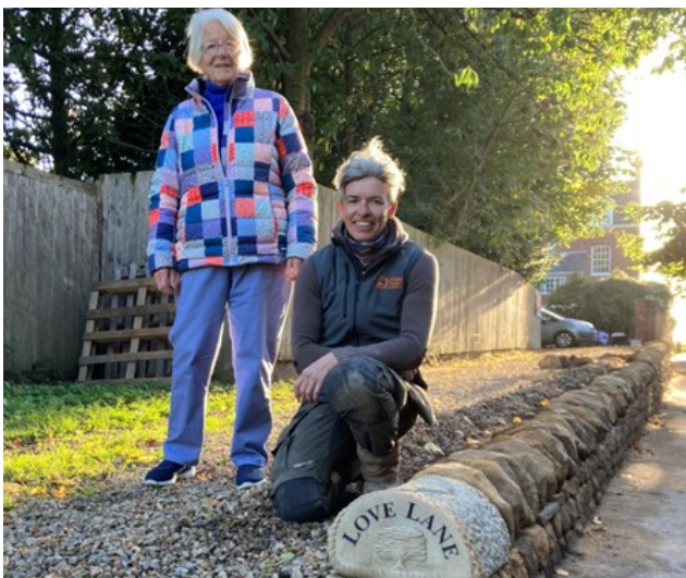
The wall completed (Emma Knowles and Barbara English)
