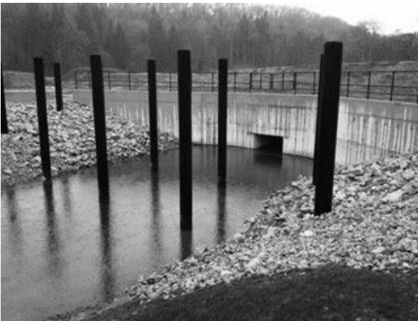
Engineered Bund (still a leaky dam) - Mike Potter
