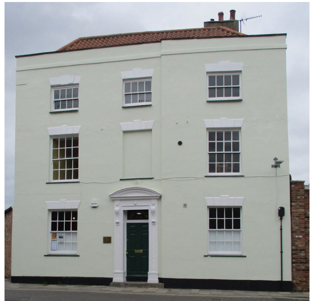
Grosvenor Club building, Walkergate
