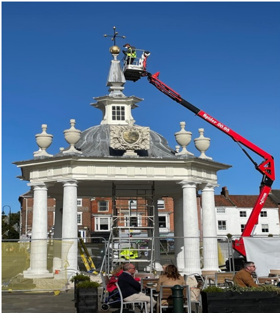
Work in progress by Pinnacle contractors
